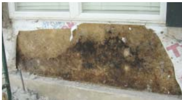
Figure 1. Where stucco (top photos) and cast stone (bottom) have been installed on the same home, the author frequently finds more severe moisture and rot damage under the cast-stone portions of the exterior. One reason is that the stucco terminates at the bottom with a weep screed, while the cast stone sits in a bed of mortar and grout, directly on a foundation ledge, with no weeps or flashings.
